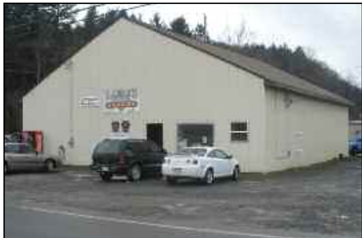
Ralph's Garage in Polk, Pennsylvania. A family-owned auto and truck repair facility since 1963.
