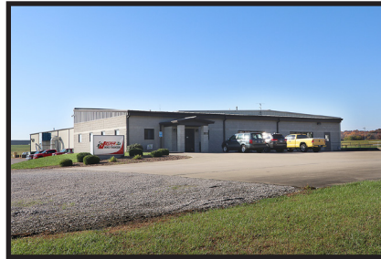
Jasper West Remanufacturing Facility
