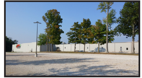
Drivetrain Remanufacturing Facility (Power Drive)
