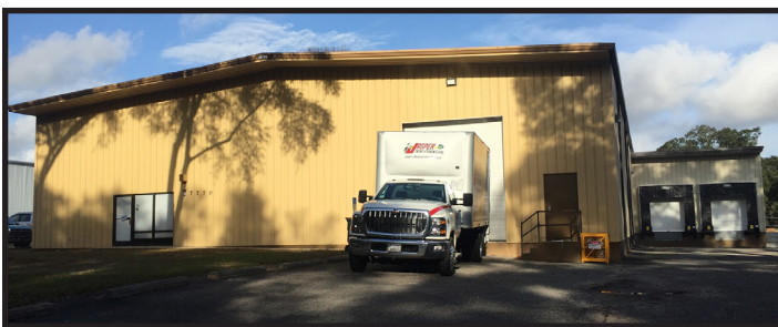
This 10,000 square foot facility in Pensacola, Florida, is JASPER's newest branch location.
