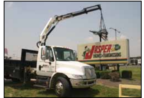
It takes a boom truck from Jasper Electric Motors, and a couple of Maintenance Associates, to position the drivetrain onto its lofty, spinning, perch.
